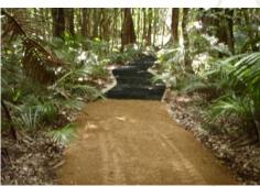
A cap layer was then applied of GAP20 with a small amount of cement added to aid compaction and surface strength.
